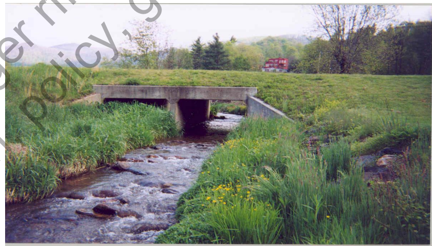
Figure 3. Culvert with Floodplain Bench
